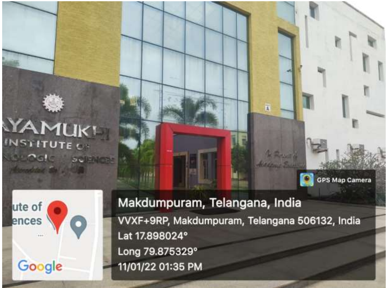
Camera Installed In Block A
