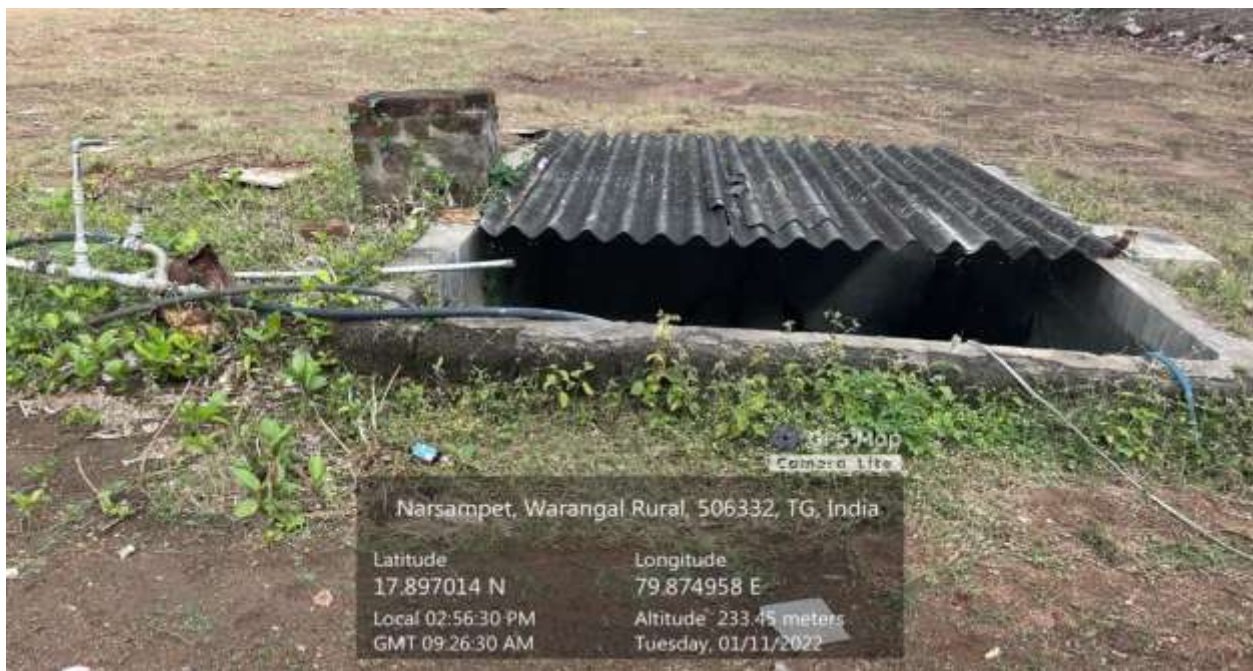
Bore wells constructed to take under ground water to supplies for usage.
