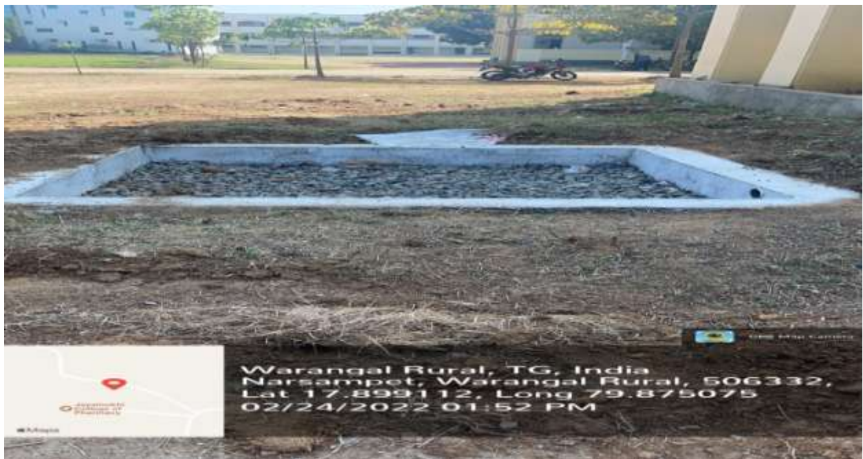
Rain water Harvesting Pits.
