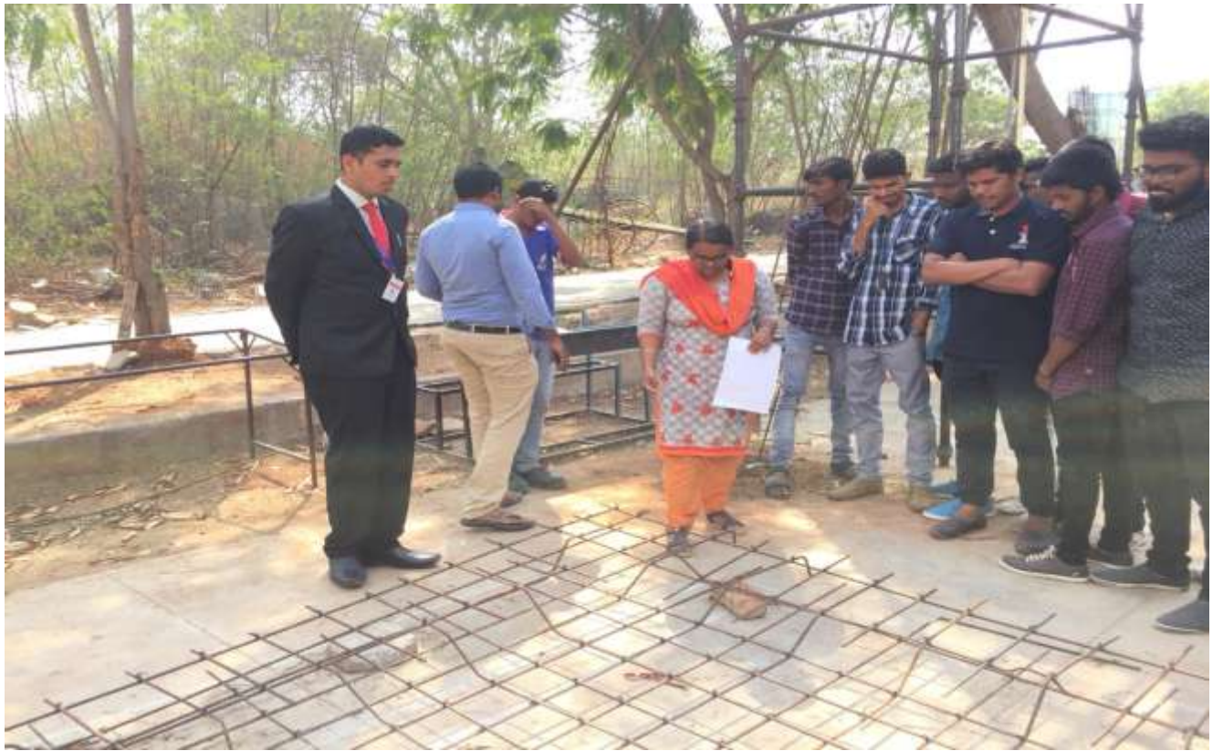
NAC Staff Explaining about Steel reinforcement in Slab
